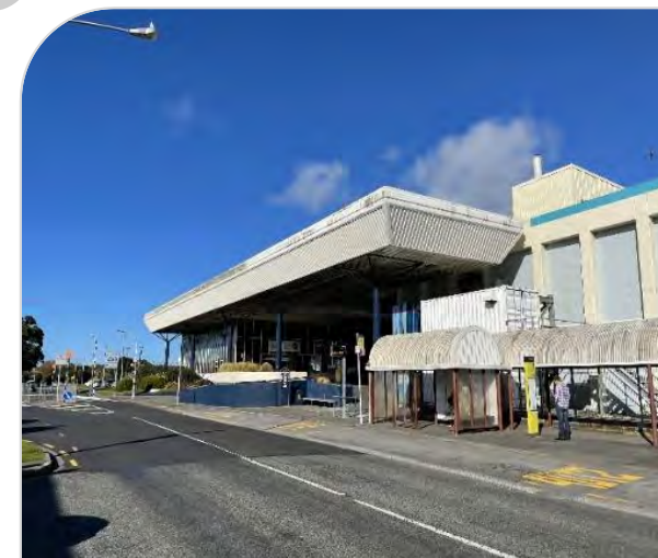
Figure 28: Main entrance on Oxford Street is disconnected from other interfaces
