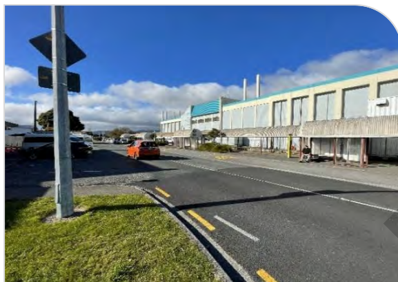
Figure 29: Oxford Terrace bus stops in front of the Wellington Water Treatment Plant
