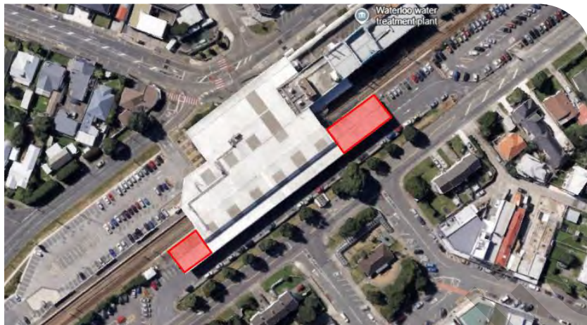
Figure 34: The areas shown in red are sections of the roof which have already been removed due to failure.
